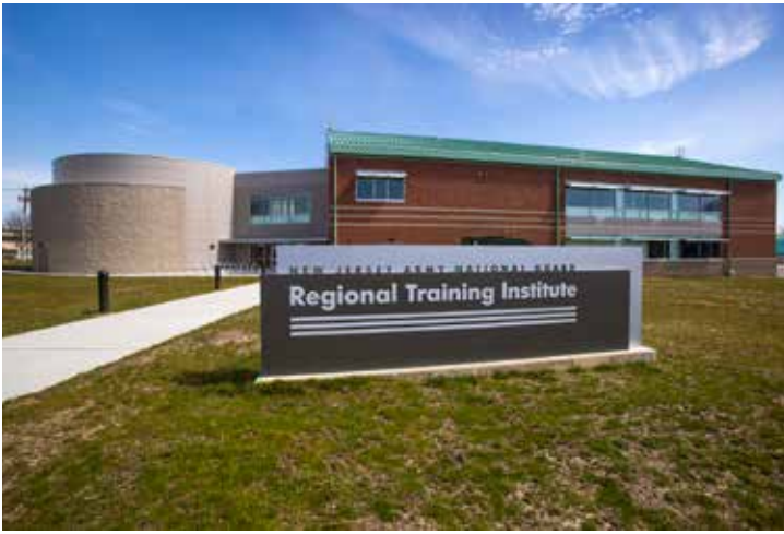
The Regional Training Institute at the National Guard Training Center, Sea Girt, N.J., April 3, 2017. The nearly $31-million dollar military construction project includes 10 state-of-the-art classrooms, an auditorium with seating for 225 students and 72 lodging rooms in the 86,000 square foot building. (NJDMAVA photo by Mark C. Olsen/Released)
